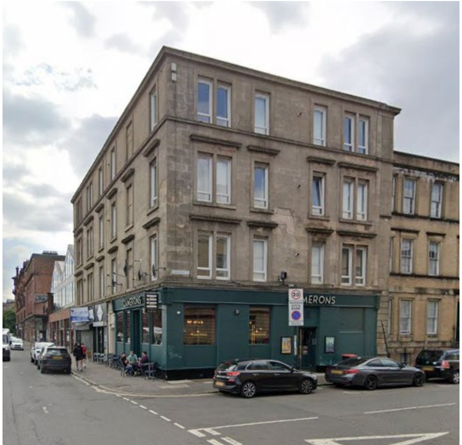
2. Carnarvon Street / St George's Road
